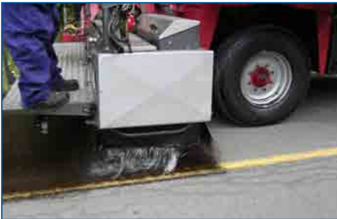
SAMI being applied to the highway surface to mitigate reflective cracking.
