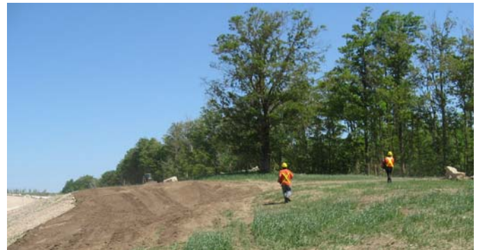
Rehabilitation efforts are underway at the east side of the quarry.
