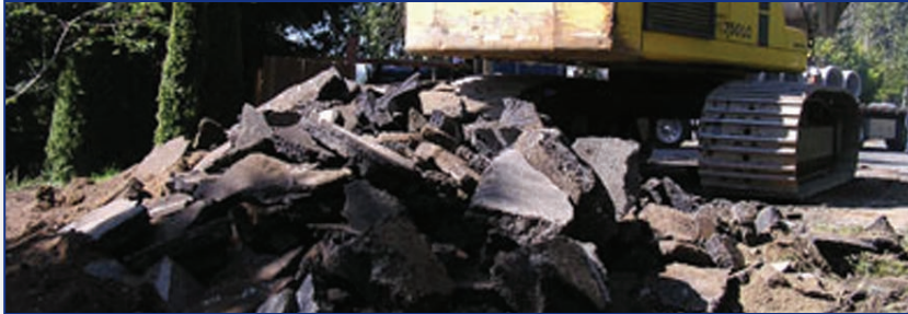
Asphalt Removal
