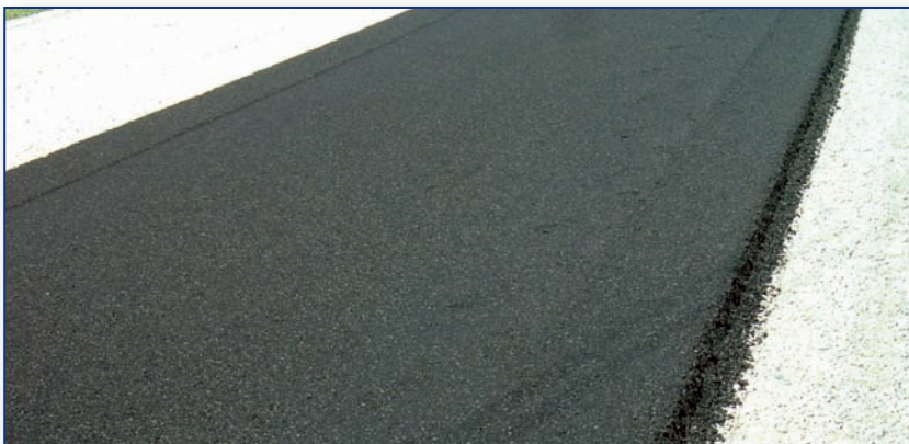
100% Cold Recycled Mix
