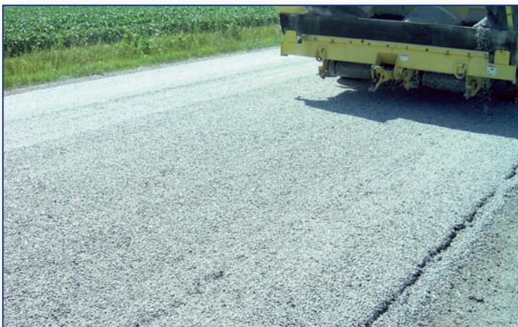
Aggregate protects FiberMat™ from traffic.
