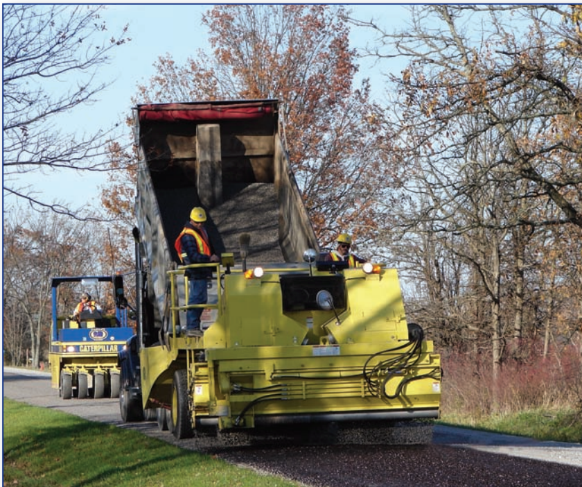
Chip Spreader and Pneumatic Roller
