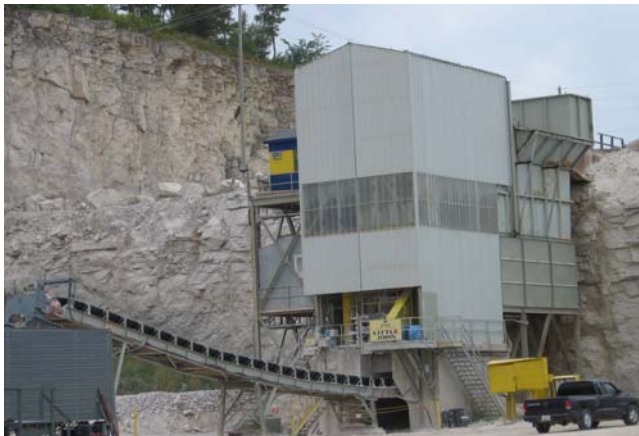
Work has been completed to enclose the primary crusher.
