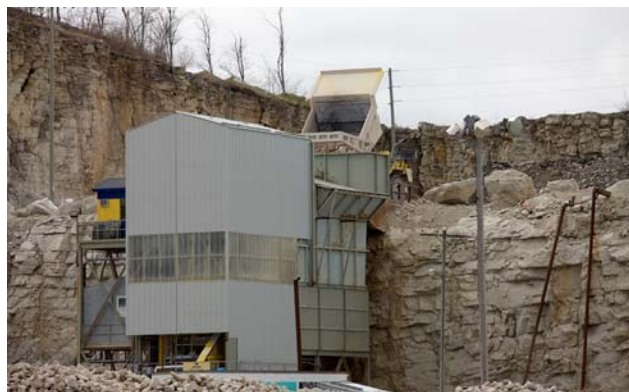
The primary crushing plant has been moved to the quarry floor and enclosed to reduce noise impacts.
