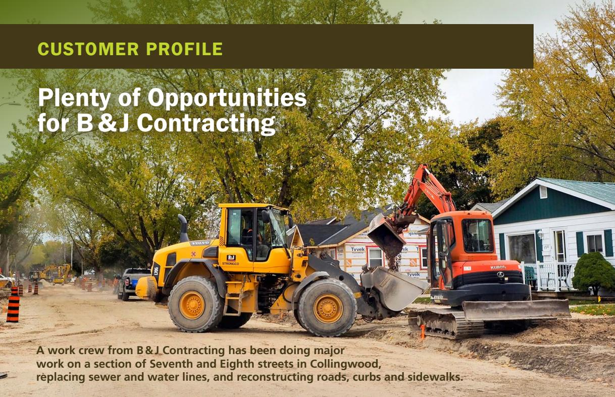
A work crew from B & J Contracting has been doing major work on a section of Seventh and Eighth streets in Collingwood, replacing sewer and water lines, and reconstructing roads, curbs and sidewalks.
